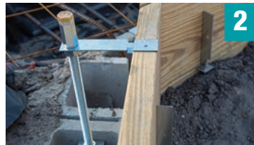
Tack Anchor Bolt Assemblies at each location
