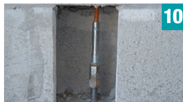
Connect each QuickTie to the anchor bolt in foundation using coupler or reduced coupler
