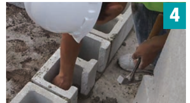
Lay CMU first course with knockouts located at each anchor bolt. (Knockouts may be placed inside or outside)
