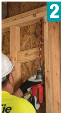
2 Drill top hole through the plate
