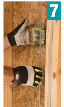
7 Check the tension on the installed cables
