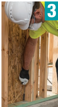
3 Blow out hole with compressed air; brush; blow again
