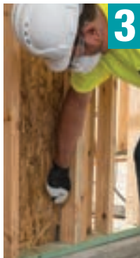
Blow out hole with compressed air; brush; blow again
