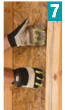
Check the tension on the installed cables
