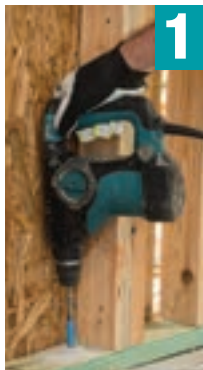
Drill bottom hole through plate and into concrete
