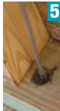
Insert proper end of QuickTie™ in epoxy and allow to cure
