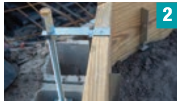
Tack Anchor Bolt Assemblies at each location
