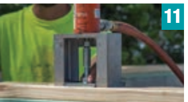
Prestress QuickTie to specified load using Masonry tension device
