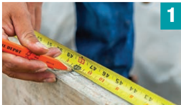
Layout QuickTie locations
