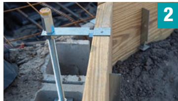
Tack Anchor Bolt Assemblies at each location
