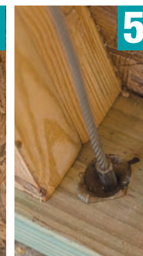
5 Insert proper end of QuickTie™ in epoxy and allow to cure
