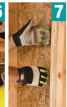
7 Check the tension on the installed cables
