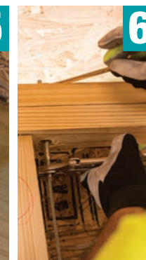
6 Tighten QuickTie™ at top plate
