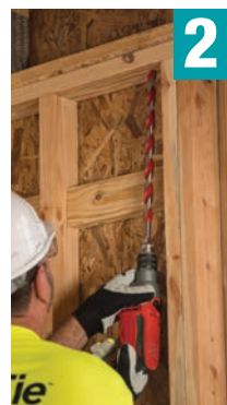
2 Drill top hole through the plate
