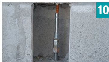
Connect each QuickTie to the anchor bolt in foundation using coupler or reduced coupler
