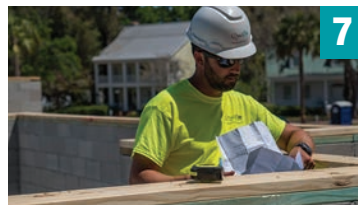
Check truss layout to ensure no conflicts with QuickTie locations
