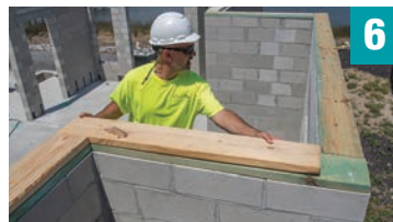
Install 2x8 Southern Pine wood top plates (pressure treated bottom plate) continuously at top of wall
