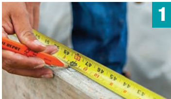
Layout QuickTie locations
