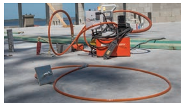
Prestress QuickTie to specified load using Masonry tension device
