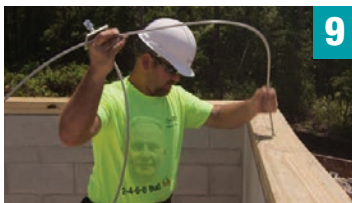
Feed QuickTie through the top plates at each anchor bolt location
