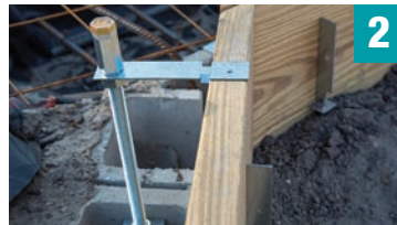
Tack Anchor Bolt Assemblies at each location
